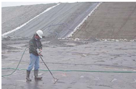
Water lance prospecting: inspection of the geomembrane surface before covering
