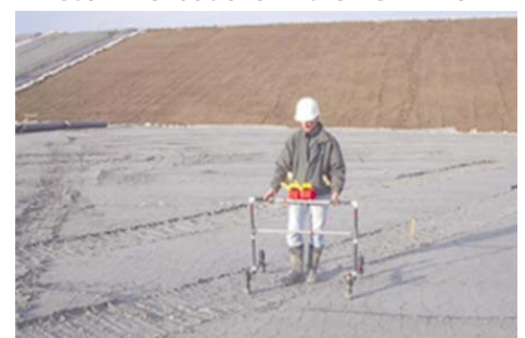
Dipole prospecting : inspection of the geomembrane surface after covering
