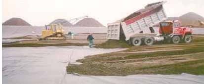
Covering of the geomembrane
