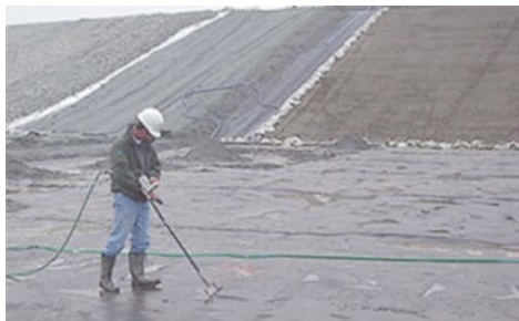
Water lance prospecting: inspection of the geomembrane surface before covering
