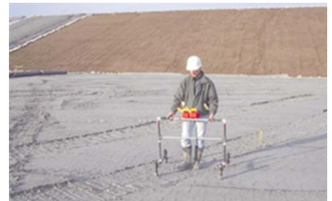
Dipole prospecting : inspection of the geomembrane surface after covering
